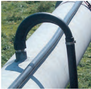
180° single gooseneck with 3/4" barb outlet shown above.
